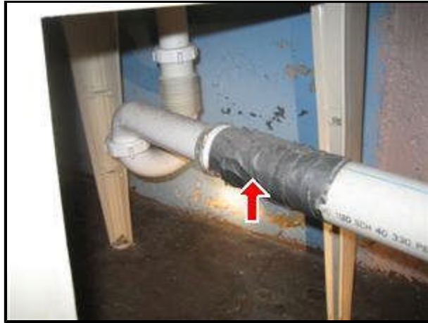
6.0 Picture 2 "Handyman" repair
